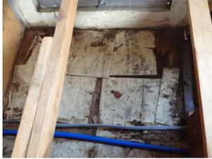
new toilet leaving a gaping area where you can see into the bumper compartment and again daylight through the floor.
